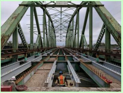
Steel repairs are complete on the historic green truss bridge on Santa Fe Avenue (US 50C), and work enters the final phase of construction.
